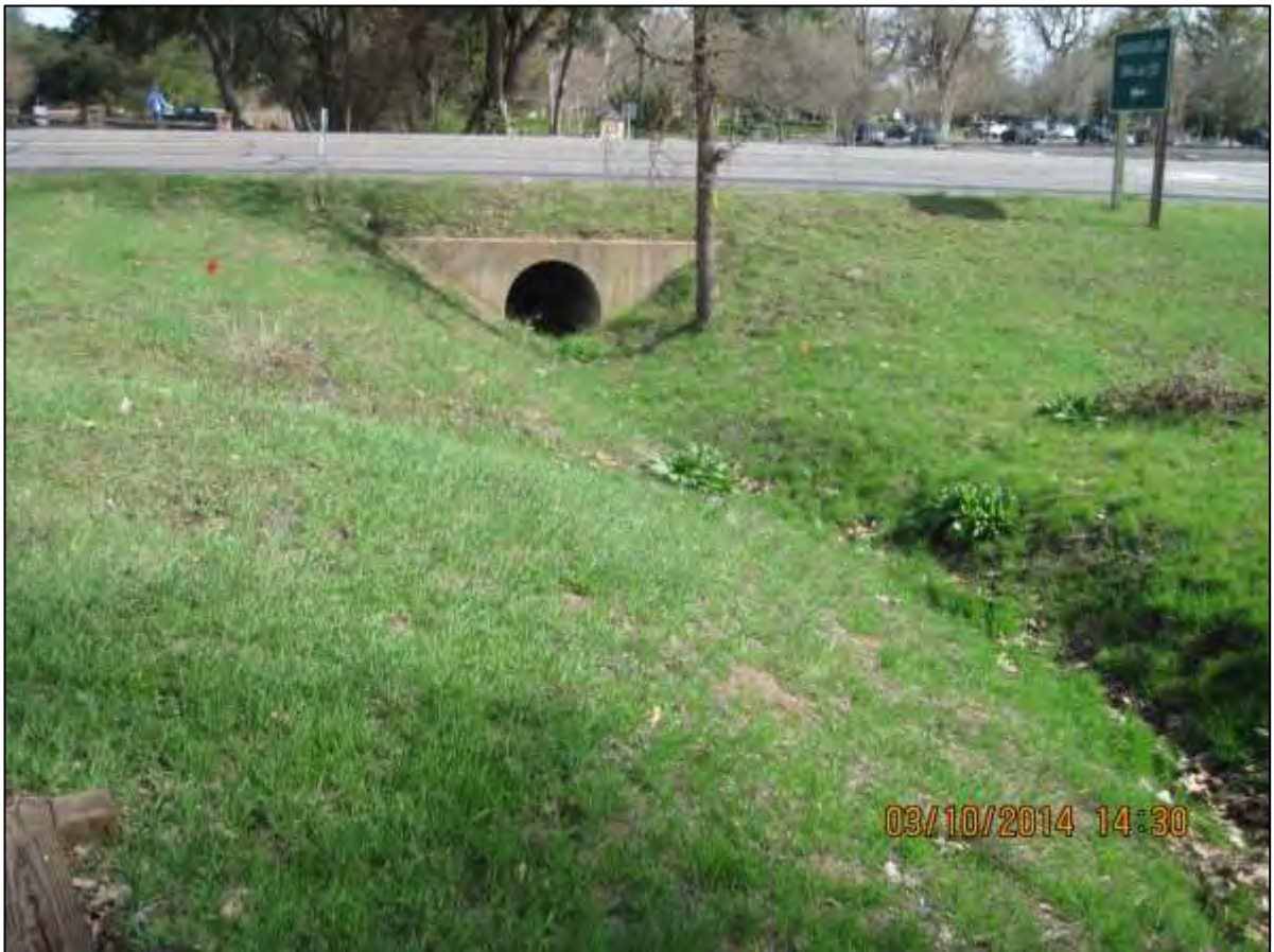
View of culvert where water enters the Atascadero Lake Park
