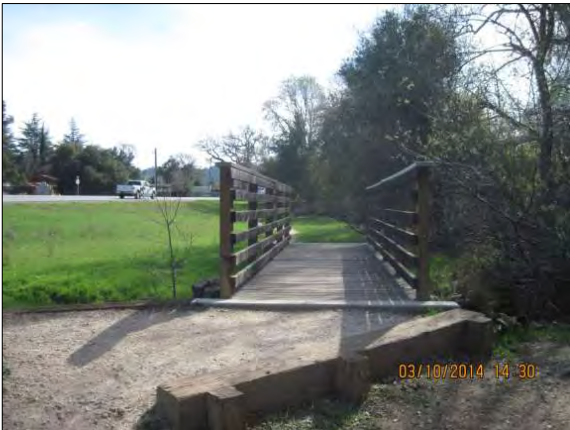
View of existing bridge over the freshwater emergent swale
