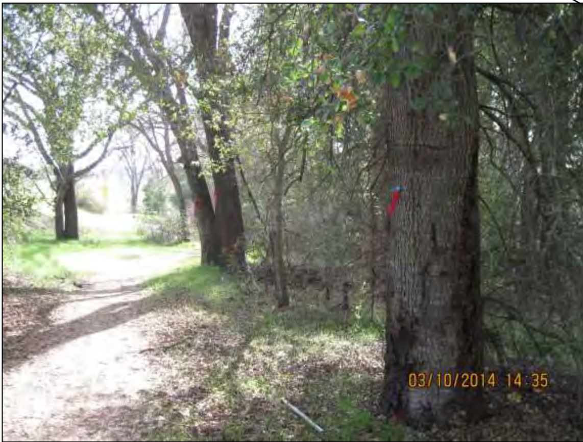
Trees that are proposed to be removed as a part of improvements to the trail.
