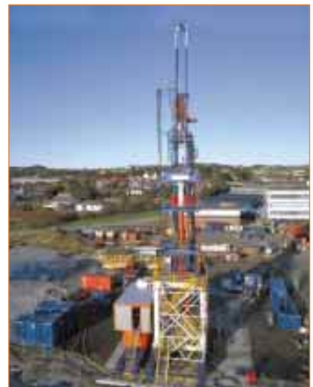
Snubbing unit Dolsnub 4 before starting work in the Norwegian sector
