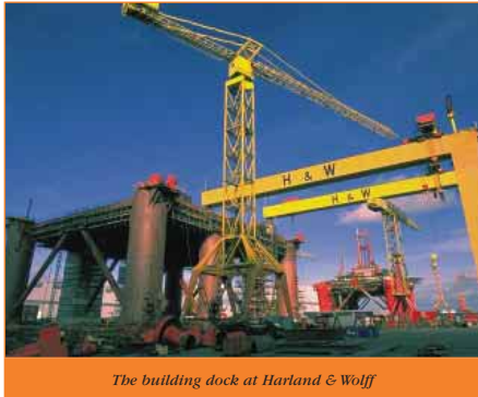
The building dock at Harland & Wolff
