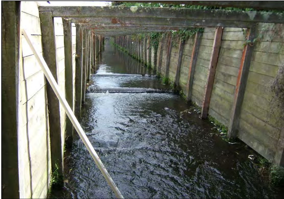
Figure 2: Horners Drain downstream from Selkirk Place
