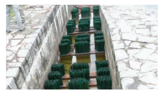
**Fig. 3.8.9.** Brush cover of the fishway bottom (Hassinger, 2002) (the Budín Weir, the Sázava River, Czech Republic, photo: J. Vait).
