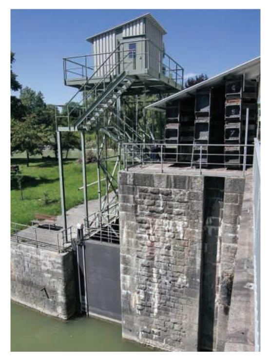
**Fig. 3.8.6.** Elevator enabling fish migrations over an obstacle. These species-selective devices ensure migration insufficiently – only at certain intervals (Wyhlen, the Rhine River, Germany, photo: M. Drahoňovský).
