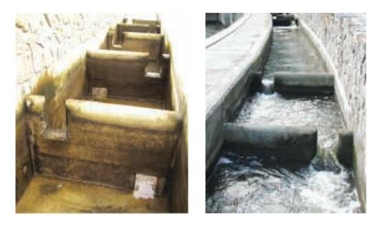
Fig. 3.8.5. An example of chamber fishway (Střekov, the Elbe River, Czech Republic, photo: Z. Vančura).
