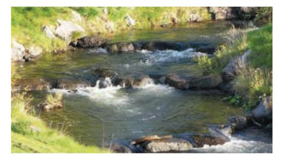
**Fig. 3.8.2.** Example of bypass channel of rock-ramp fishway – in detail (Obermaubach, the Rur River, Germany, photo: M. Drahoňovský).
