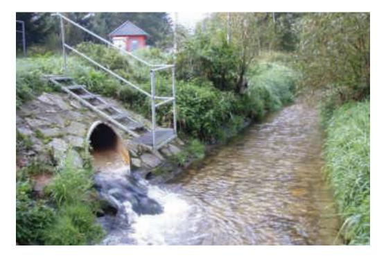
**Fig. 5.5.8.** Pipe inlet of treated municipal waste waters from the Prachatice sewage treatment plant into the **Živný Brook.** These waters represent approximately 30% of the recipient flow-rate. Fish occurring under this STP show reproduction disorders as well as other significant physiological changes in organisms (photo: T. Randák)
