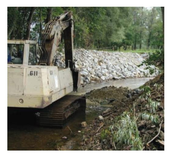
**Fig. 4.6.7.** Common destruction method of a river bed as part of the so-called anti-flood modifications (photo: T. Randák).
