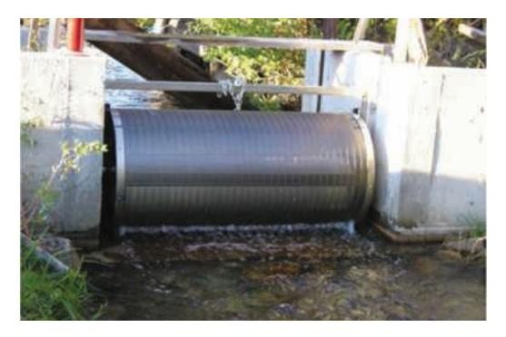
**Fig. 5.3.8.** Wedge wire screen cylinder (photo taken from http://www.bdiscreens.com/fishdiversion.htm and used with the agreement of B. Deo-Volente, Inc. 1255 Monmouth Blvd., Galesburg, Illinois 61401).
