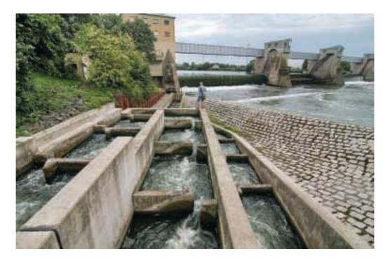
Fig. 3.8.3. Vertical slot fishway (Ladenburg, the Neckar River, Germany, photo: M. Drahoňovský).
