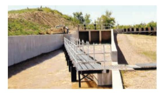
**Fig. 5.3.6.** View of the stream of the irrigation channel – inclined position of the barrier – Louver (photo taken from http://www.usbr.gov/pmts/hydraulics\_lab/pubs/manuals/fishprotection/ used with the agreement of the U.S. Department of the Interior Bureau of Reclamation Denver, Colorado 2006: Fish Protection at Water Diversions, A Guide for Planning and Designing Fish Exclusion Facilities 2006, pp. 480).
