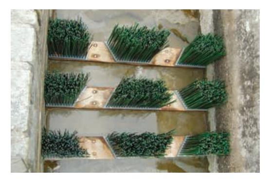
Fig. 3.8.10. Details of brushes in the fishway in the Sázava River (photo: J. Vait).
