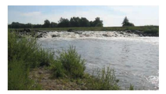
Fig. 5.2.3. Riprap weir on the Morava River near Lanžhot (photo: Z. Adámek).
