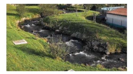
**Fig. 3.8.1. Example of the bypass channel of the rock-ramp fishway – the complete view** (Obermaubach, the Rur River, Germany, photo: D. Bůžek).
