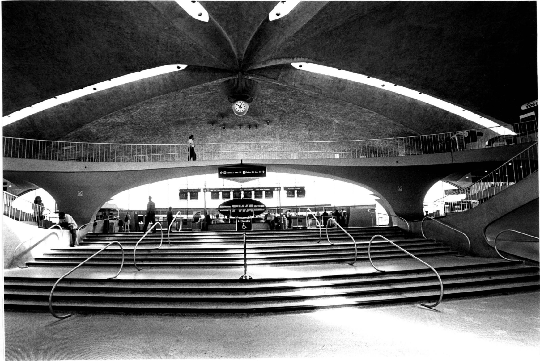
Trans World Airlines Flight Center at New York International Airport Interior. TWA Flight Center Interior, John F. Kennedy International Airport, Queens Central area of main terminal.
