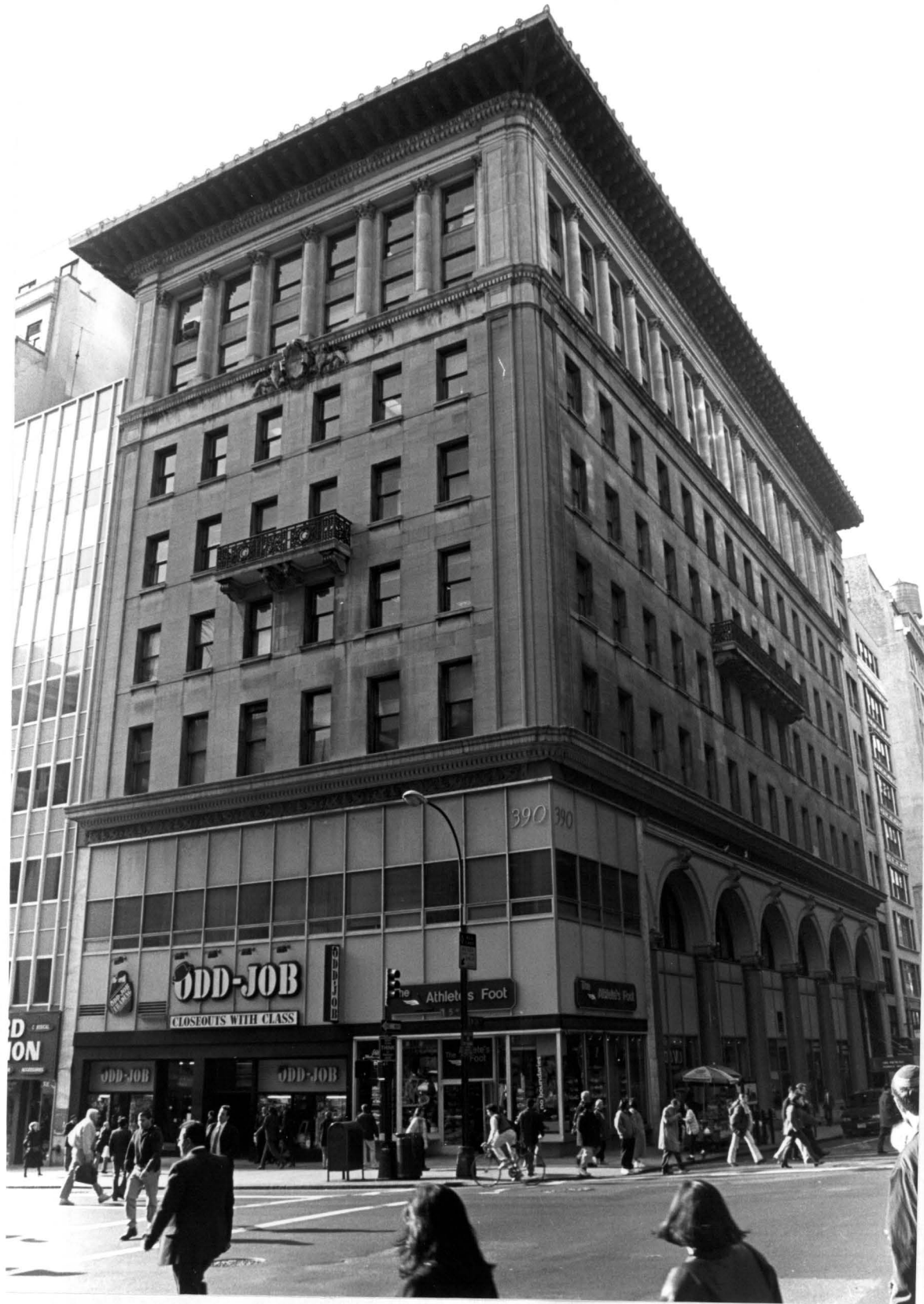
Gorham Building, 390 Fifth Avenue, aka 386-390 Fifth Avenue and 2-6 West 36th Street, Manhattan Photo: Carl Forster
