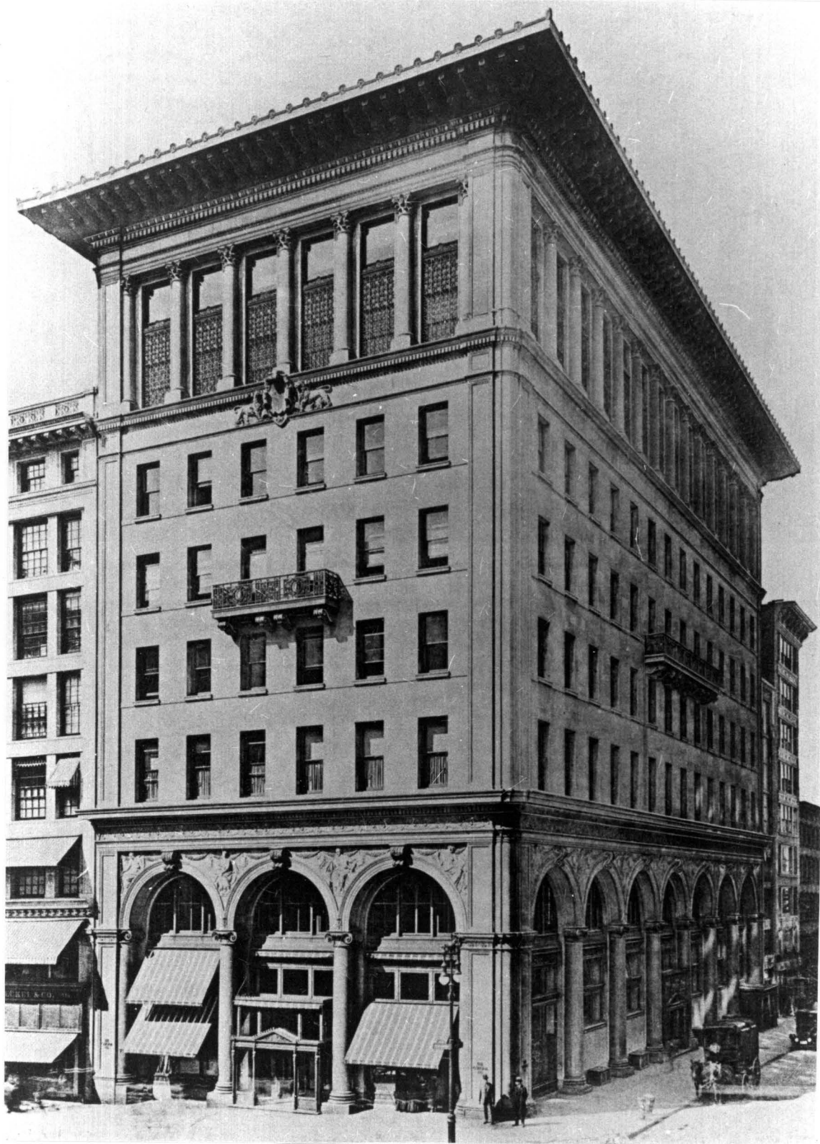
Building for the Gorham Company, New York City Source: A Monograph of the Work of McKim, Mead & White, 1879-1915 , pl. 234
