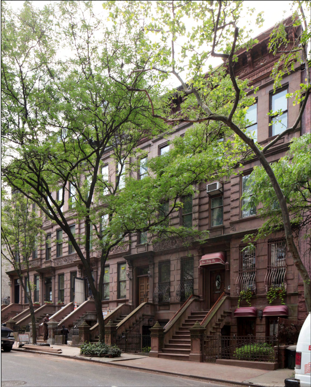
Figure 9 258 to 266 West 71 st Street (M. V. B. Ferdon, 1892) Photo: Christopher D. Brazee, 2013
