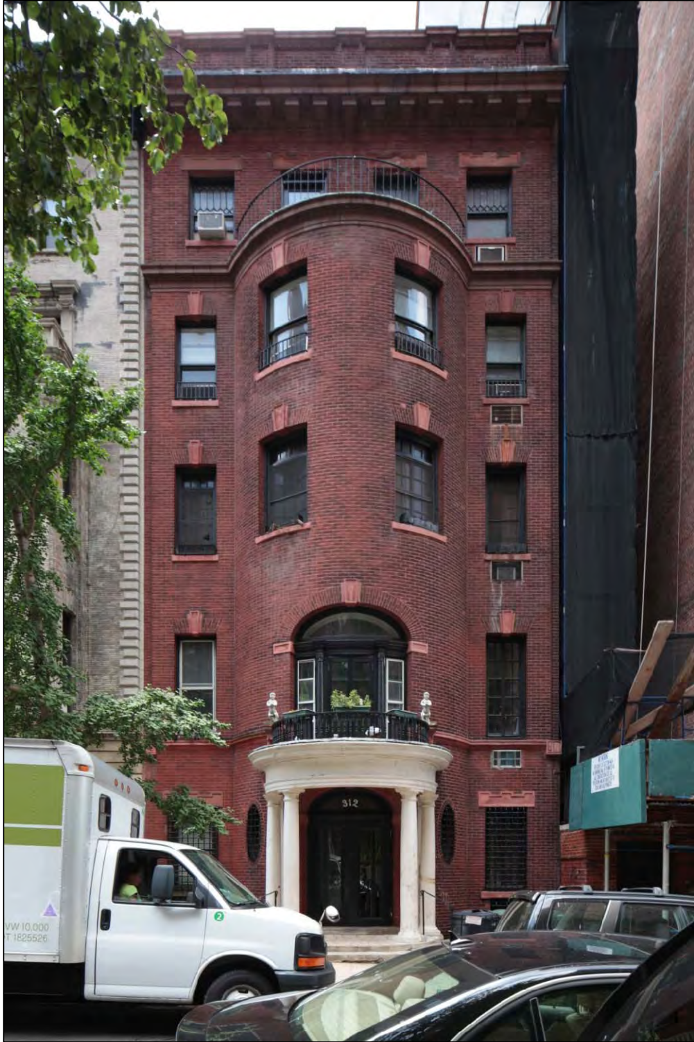
Figure 10 312 West 73 rd Street (C. P. H. Gilbert, 1897-98) Photo: Christopher D. Brazee, 2013
