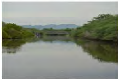
2. Bridge at Brampton
