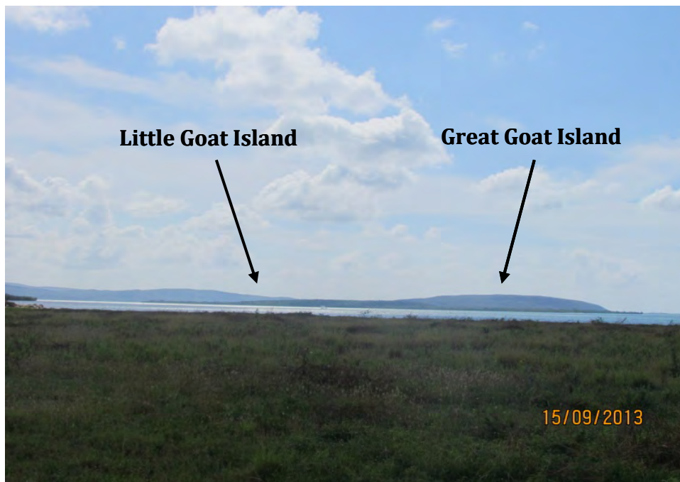
Plate 73: Goat Islands (background) as seen east of main access road to JPSCo's Old Harbour Bay Power Plant
