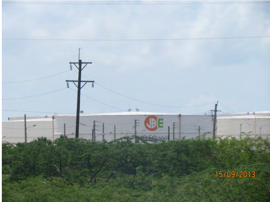
Plate 75: Jamaica Broilers Ethanol Plant
