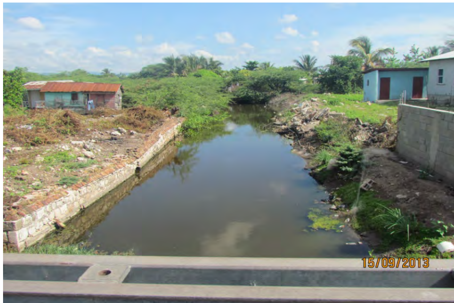
Plate 71: Major Culvert through Old Harbour Bay Fishing Village
