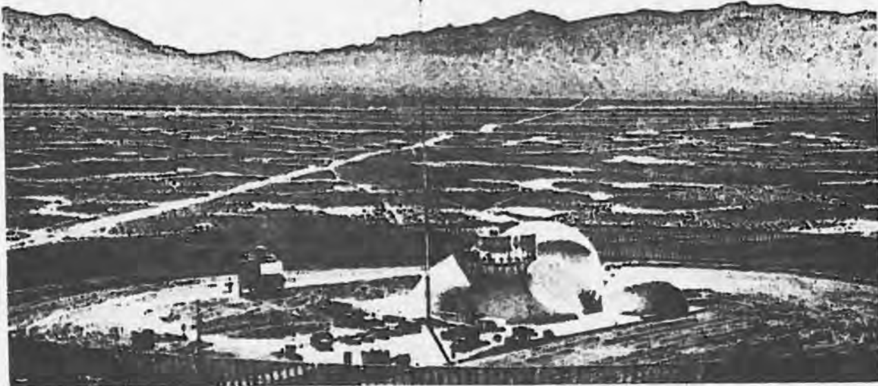
"TEST VERSION OF MULTI-FUNCTION ARRAY RADAR (MAR), under development at White Sands Missile Range (WSMR), New Mexico, is expected to provide for defense against long range ballistic missiles. Large dome contains MAR receiver equipment and smaller domes house the transmitters." (Army R&D September 1964)
