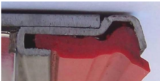
Figure 2: Wiper sealing gap between cover segments.
