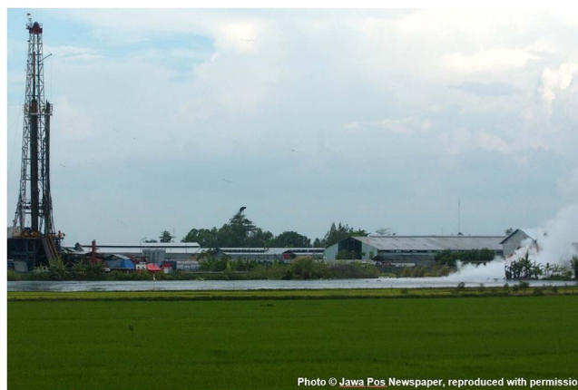
Fig. 7. Photo of the TMMJ drill rig and BJP-1 location and the first documented Lusi eruption site approximately 100 m from the well (“40ft SW of flare pit”). Exact time of the photograph is not documented, but is within the first 3 days of the Lusi eruption, as the drill pipe is clearly still visible in the racks on the rig tower, and daily drilling reports note that this was removed before sunrise on the 2nd of June. Photo from Guslan Gumilang/Jawa Pos, with permission.
