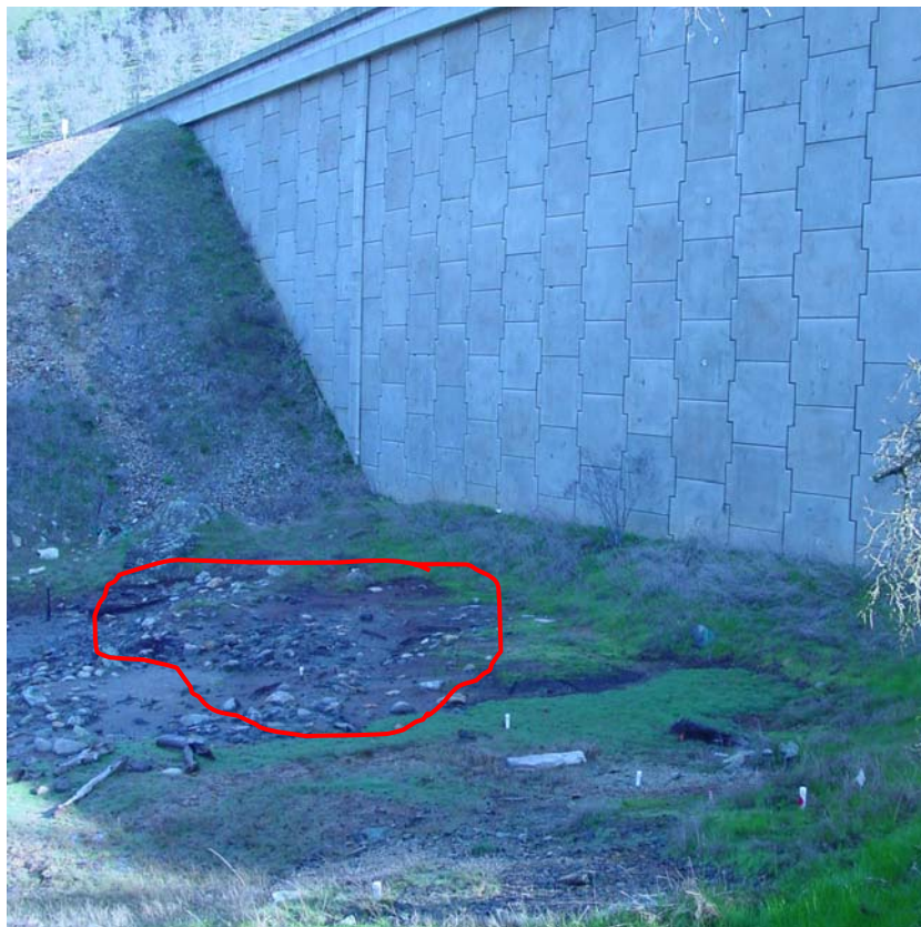
Figure 14 Potential fill removal area in Spring 3.
