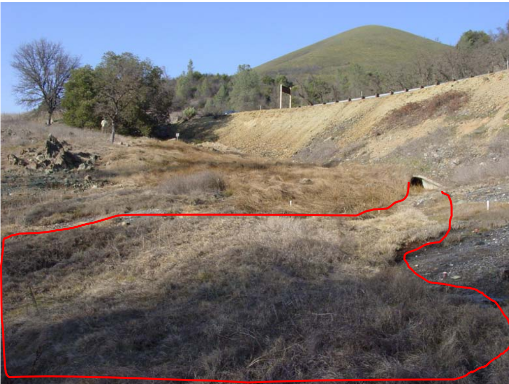
Figure 9. Looking north toward the highway in Spring 2. The alluvial fan and fresh water plume formed by the culvert stream is bounded by the red line.
