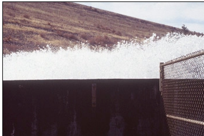
Aerator at the Mokelumne Hatchery
