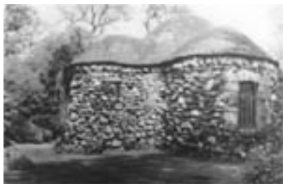
Outside view of Shell House, Curraghmore
