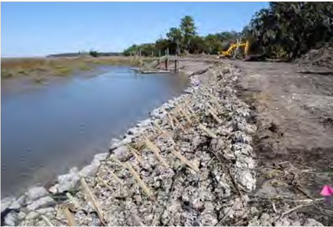
Figure 4. Living shoreline using vegetation and edging on Sapelo Island, Georgia
