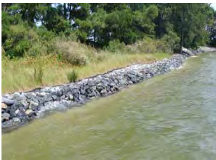
Figure 3. Example of use of marsh toe revetment in a living shoreline
