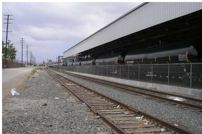
Ethanol Tank Train Transfer Facility at Watson Yard
