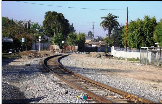
El Segundo Industrial Lead at 109th Street
