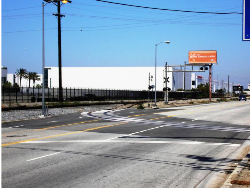
Torrance Industrial Lead at 204 th Street paralleling Normandie Avenue
