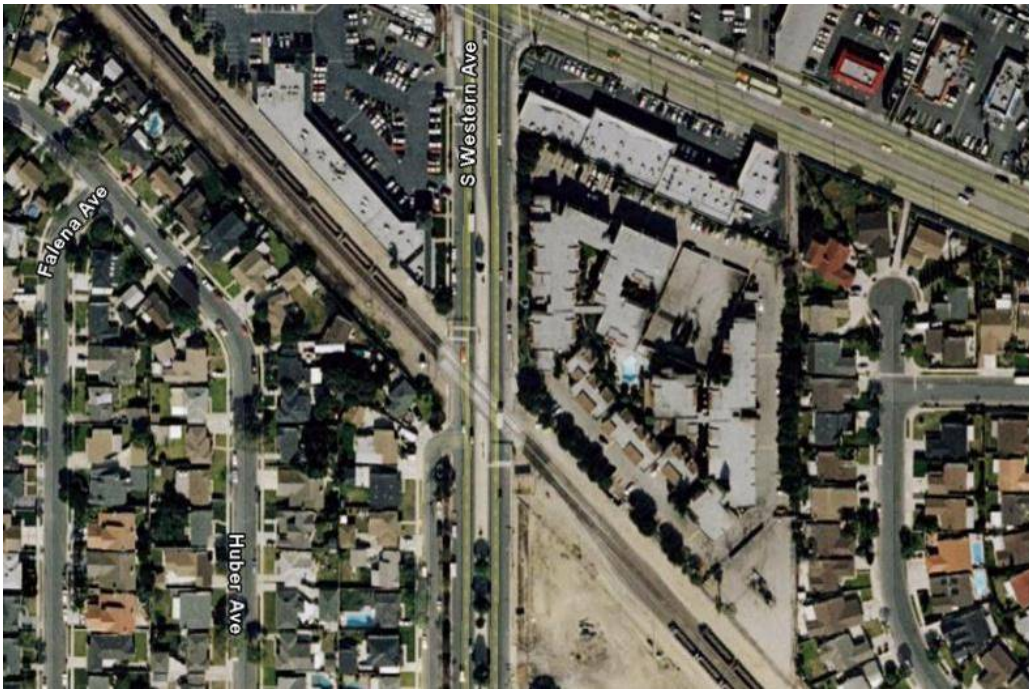
BNSF Grade Crossing Western South of Sepulveda
