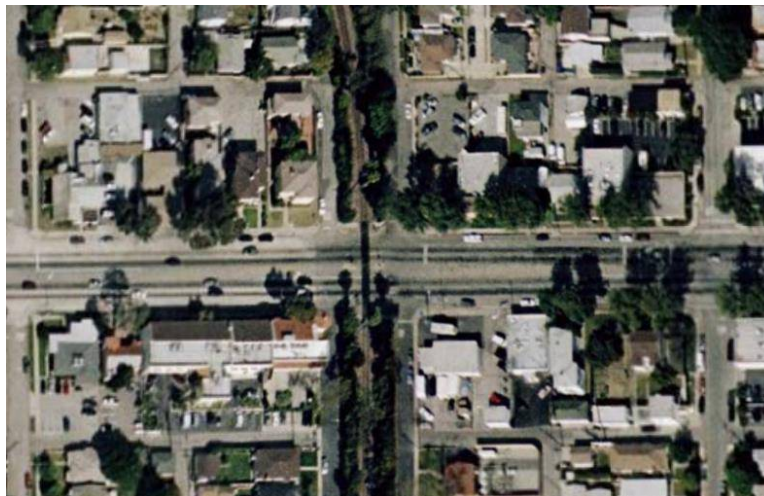
BNSF Grade Crossing Torrance East of Crenshaw
