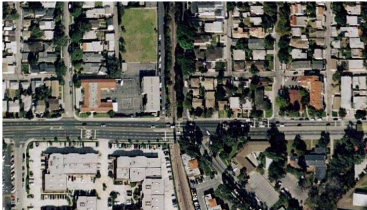
BNSF Grade Crossing Carson East of Crenshaw
