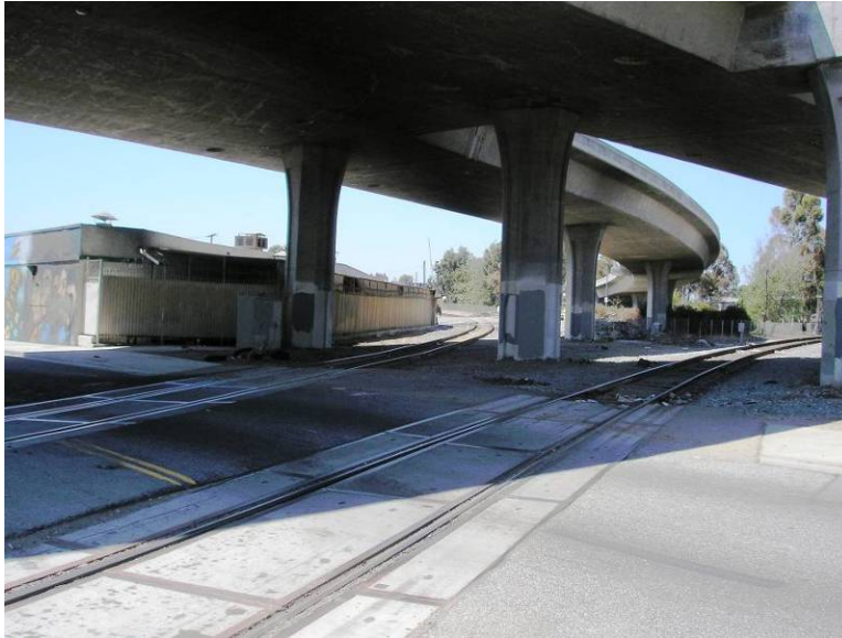
El Segundo & Torrance Industrial Leads at South Broadway looking west
