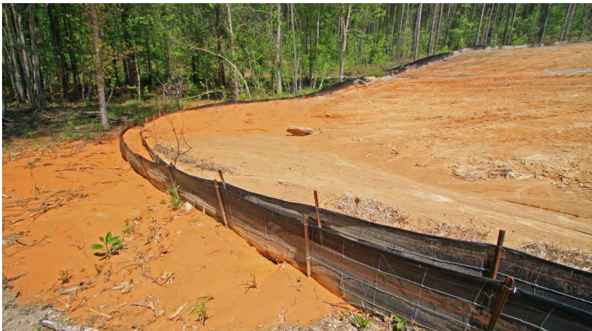
Figure 3-21. Failed erosion control at road construction site
