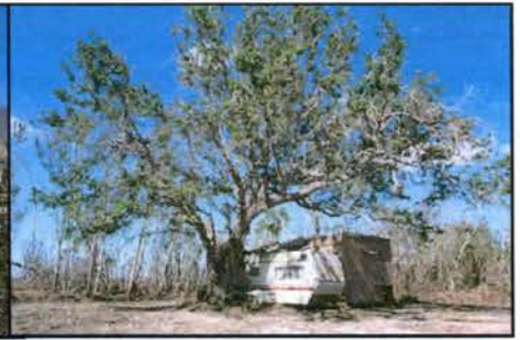
Homesite on Little Chenier after Hurricane Rita. Live oak tree provided some protection for summer-camp trailer (April 8, 2006)
