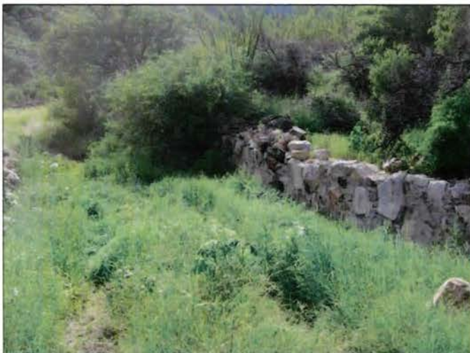
Path to collecting site - wall where the water was pouring over that made the path impassable.
