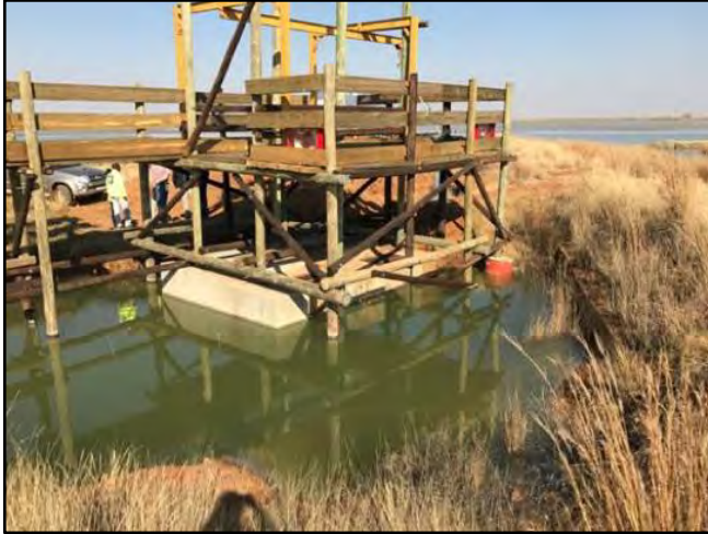
Plate 2.2: Example of Traditional Penstock Decant System
