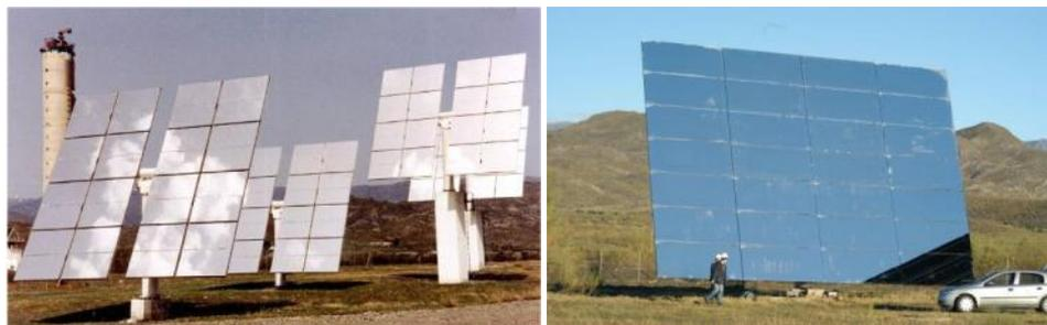
**Figure 8: Opened T structure with complete turn down position (left) and Closed T structure without complete turn down position (right). (Source: Kolb2007)**
