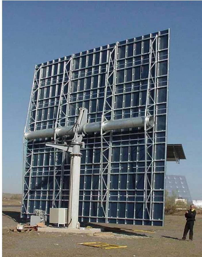
**Figure 6. Heliostat with pedestal and frame assembly (Source: PSA)**
