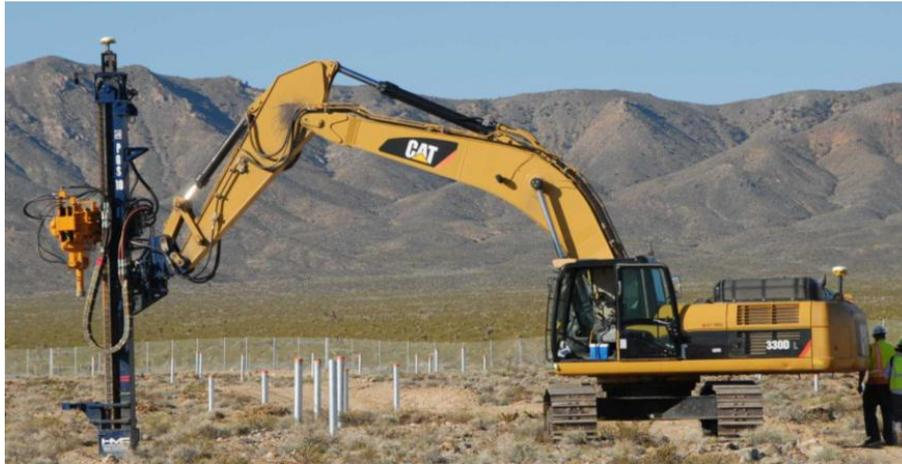
**Figure 5. Pylon insertion at Ivanpah (Source: BrightSource)**
