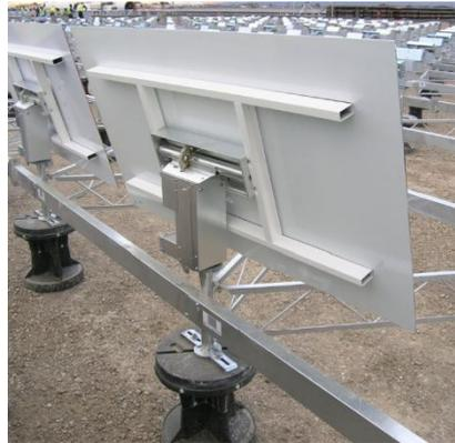
**Figure 7: Low cost support structure for small heliostats (Source: eSolar)**
