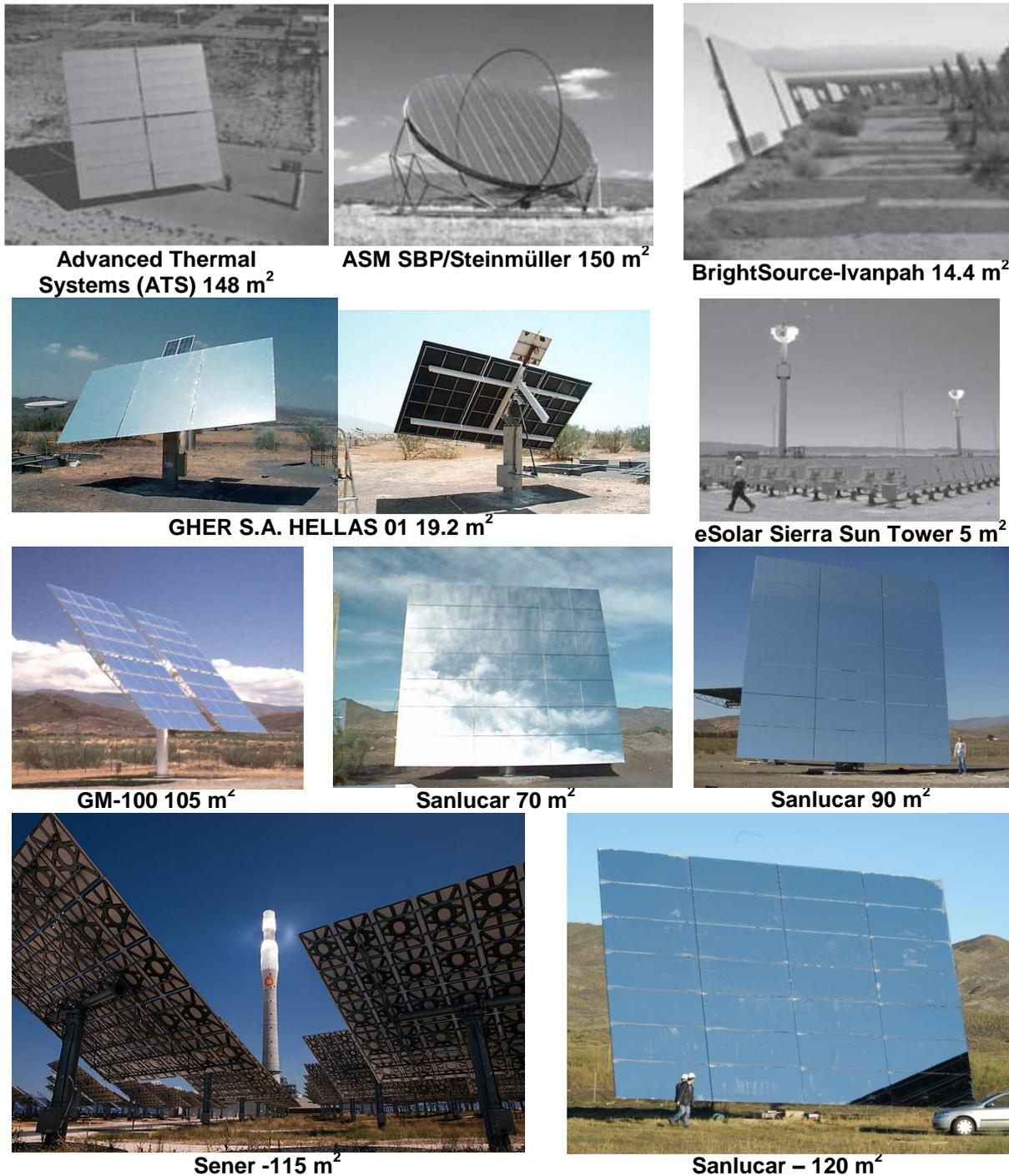
**Figure 1: Representative heliostat designs and sizes (adapted from [Kolb et al., 2007]).**
