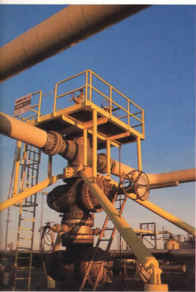
Left, Unit 3's cooling tower. Top, an Imperial District employee uses a scale model to explain the plant's operation to guests at the April dedication. Above, the wellhead of Vonderahe 1, the world's largest geothermal well.
