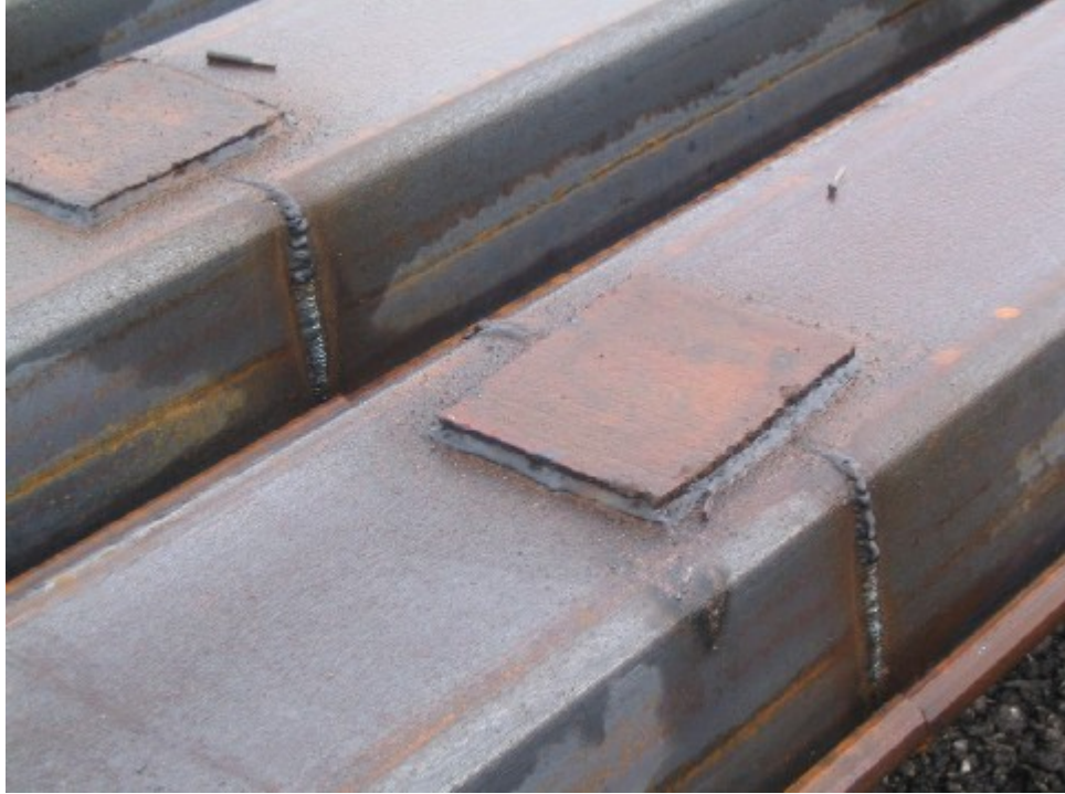
Close view of the sheet pile splicing
