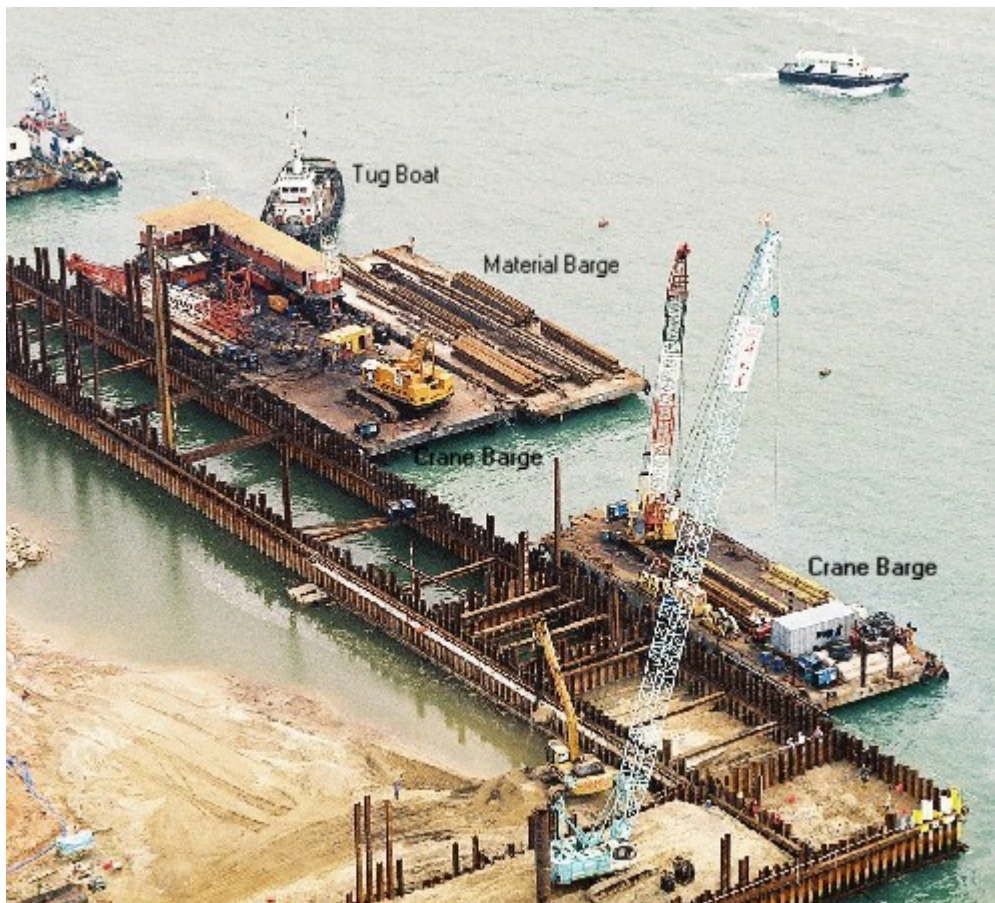
A typical layout when piling for marine sheet piles
