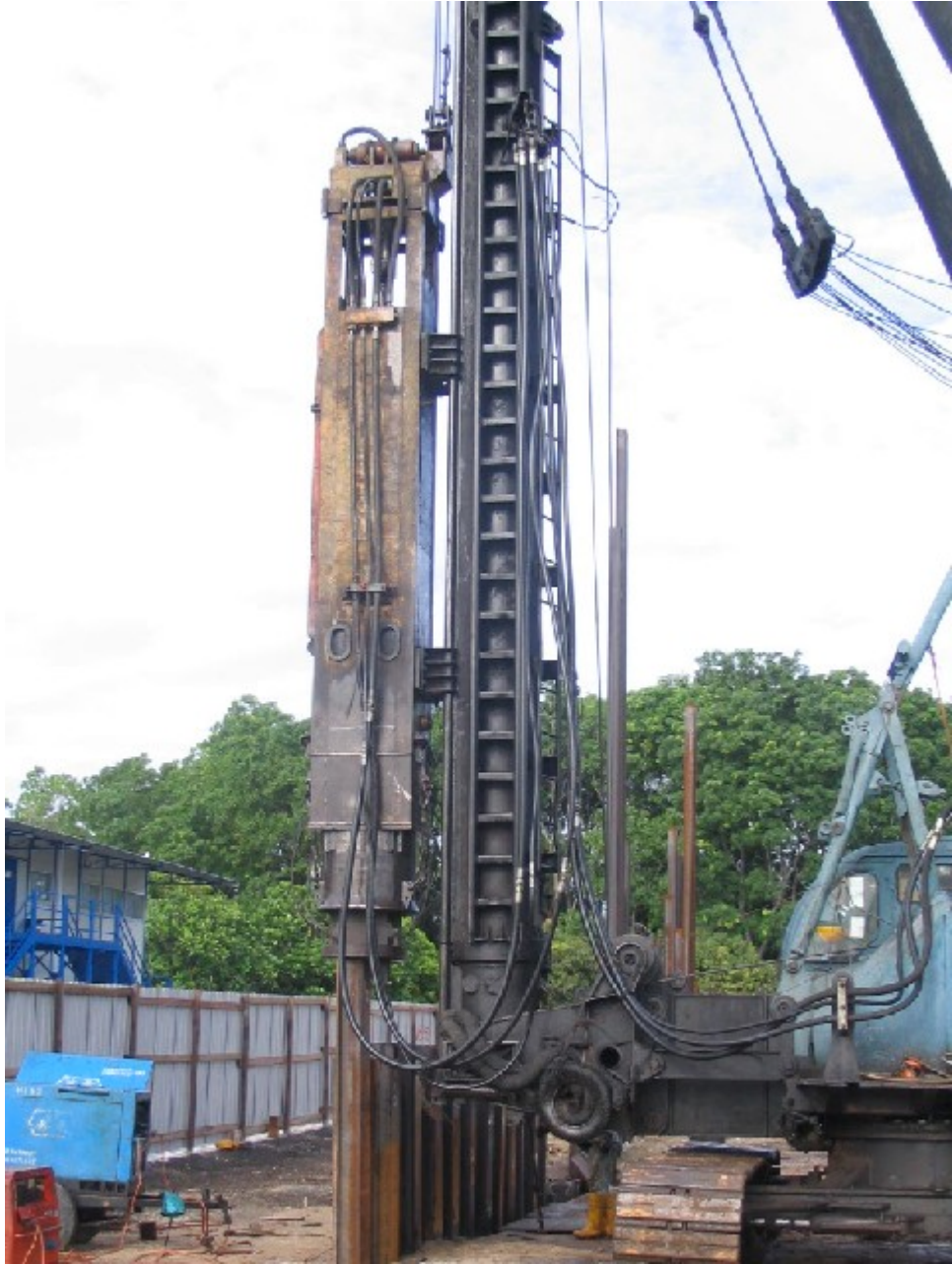
Impact Hammer Driving: A 7-ton hydraulic hammer
