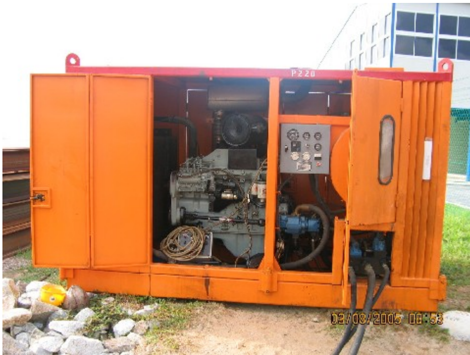
Vibro-driving: Power pack for vibro hammer
