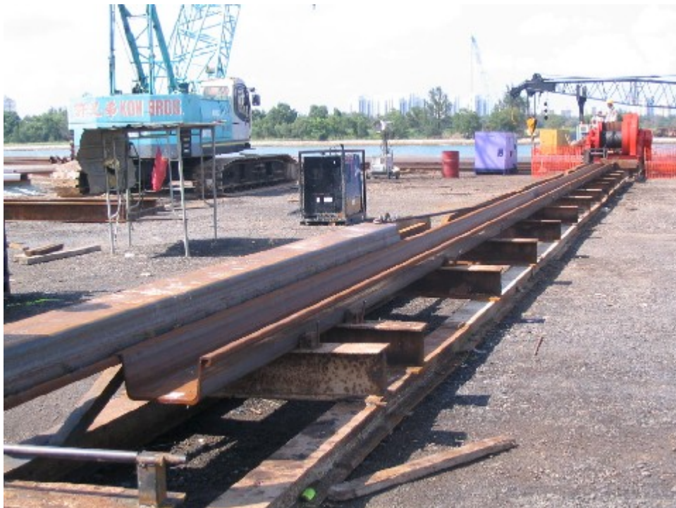
Interlocking 2 pieces of sheet piles to become a pair
