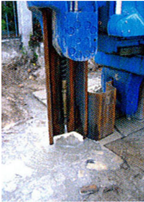
Left: Water jet; Right: Pre-drilling
