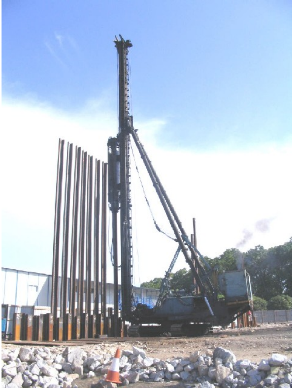
Driving sheet pile using hydraulic hammer
