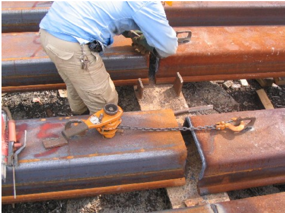
Welding of splicing
