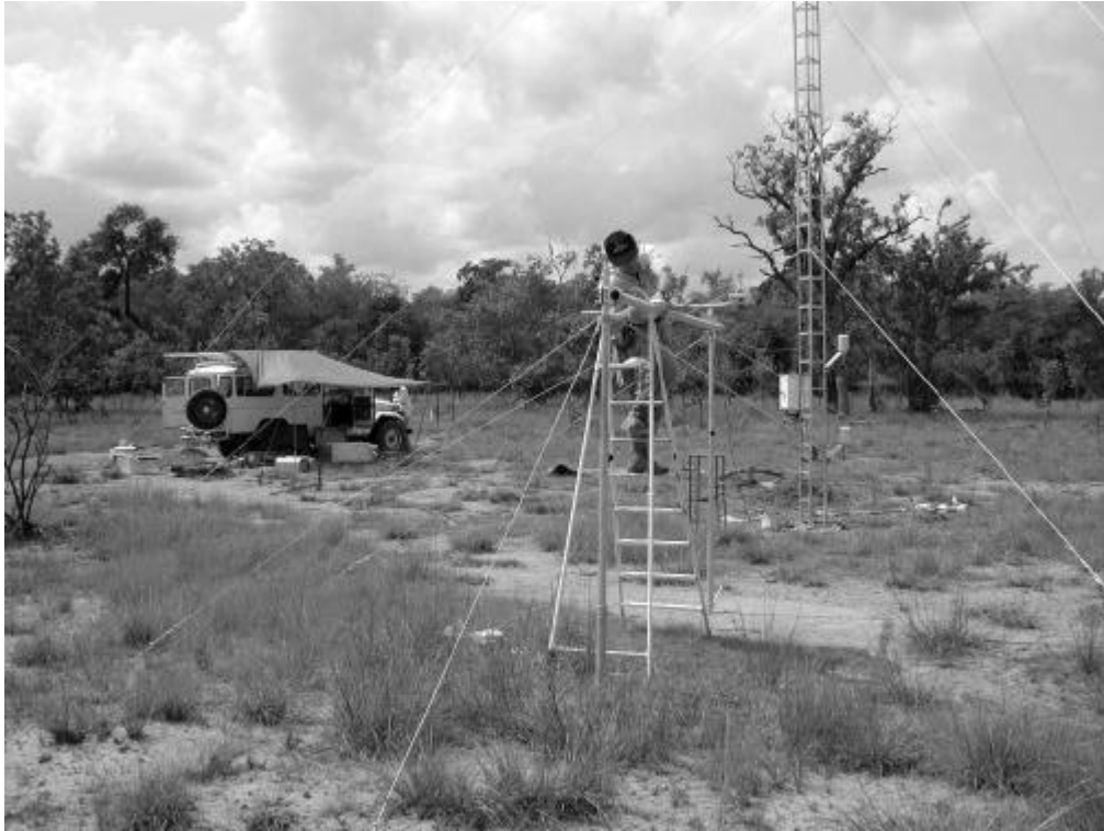
Fig. 1: Installation of technical equipment at the savanna station
