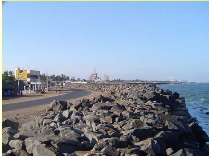
Fig. 4.3 Groynes for coastal protection adjoining Ennore Expressway
