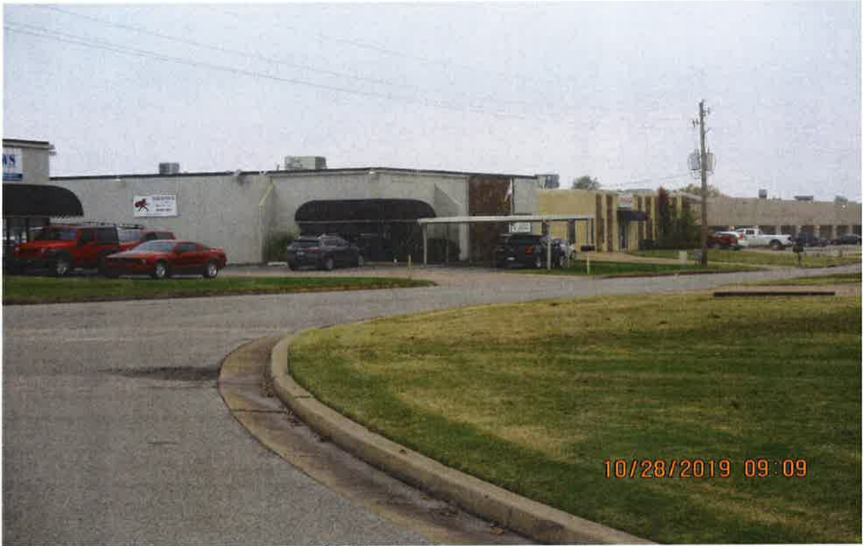
View facing Northwest on 94 th E. Ave.
