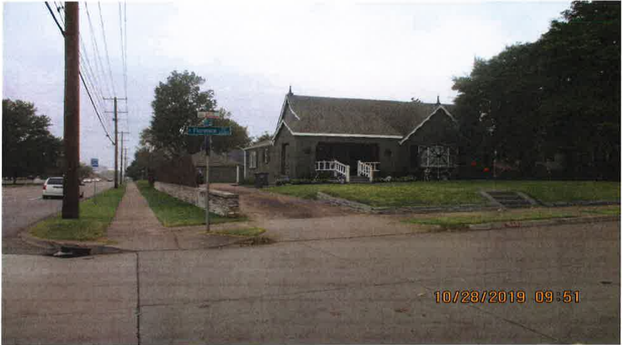
Subject property facing West
