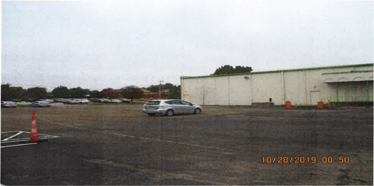
Rear of Subject property
