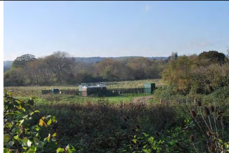
Photo 2. Sewage works within valley floor
