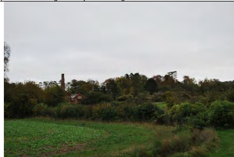
Photo 4. Twyford Pumping Station which is a distinctive landmark
