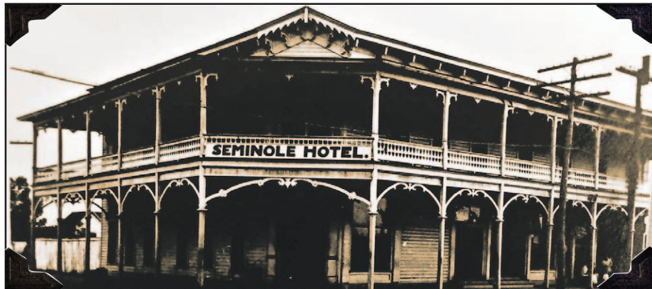
The Seminole Hotel built in 1887 as Dade Hotel at Marion Avenue and Taylor Street.
