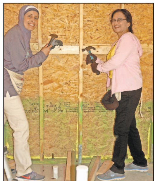
Samera Musallet and Haleema Moopen work on a wall.
