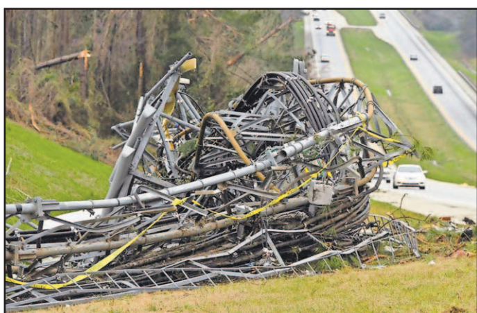
A huge cell tower destroyed by the tornado in Smith's Station, Alabama.
