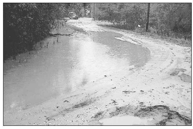
Carter and Colby streets off Central Avenue between State Road 44 and Forest Drive, have become safety and health hazards when it rains. The Inverness city council met with residents at an assessment workshop Thursday.
