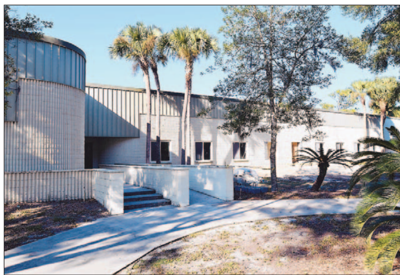
The county is relocating offices to the Meadowcrest area by January.
