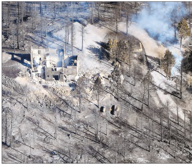
This aerial photo shows a home completely burned Tuesday during the Lower North Fork Wildfire near Denver.
