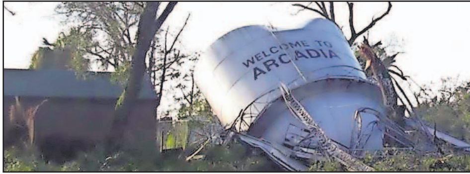
This tumbled water tower made national news.
