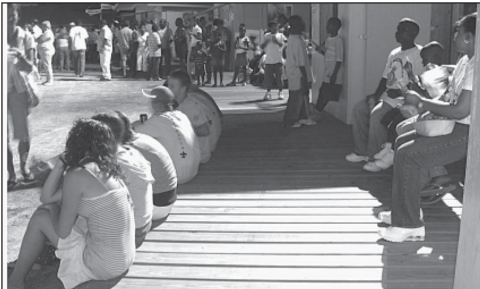
A boardwalk now joins the booths at Goombay Park in Marsh Harbour. The Abaco Club on Winding Bay provided the materials while the Marsh Harbour Town Committee provided the labour. It makes much more seating for the crowds who attend events there. Picnic tables are between most booths.
