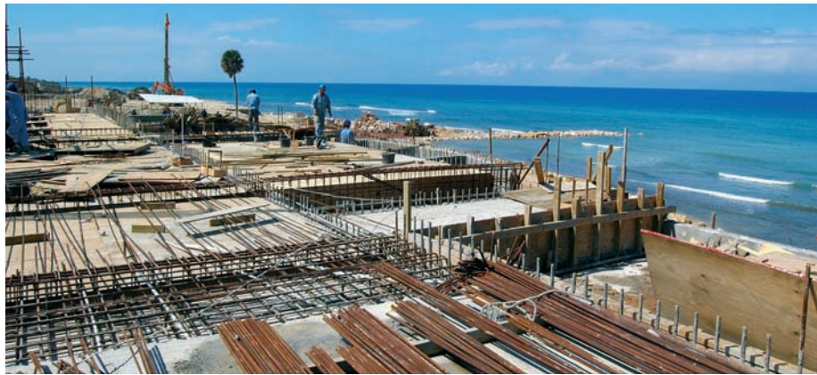
Construction is moving ahead at the Palmyra Resort & Spa
