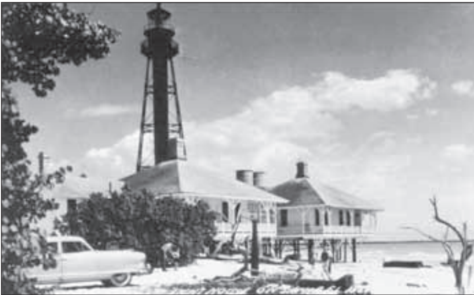
In this postcard depicting the Sanibel Lighthouse, circa early 1960s, heavy erosion allowed the lighthouse keepers to fish directly from the porch of Quarters No. 2
