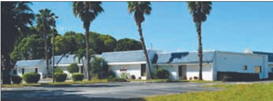
PACE Center For Girls new building at 3800 Evans Avenue, Fort Myers
