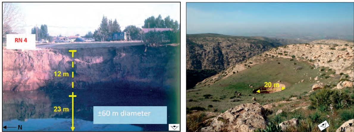
Figure 5: The 2 major sinkholes in the study area. Left: the 1988 RN4 sinkhole in the Chelif Basin 500 m from the carbonate piedmont (Photo taken by Pr. Mostefa GUENDOOUZ on 16/06/1988). Water table is 12 m below the level of the road. Right: The Bir Djeneb in the carbonate Ouarsenis Mts.
