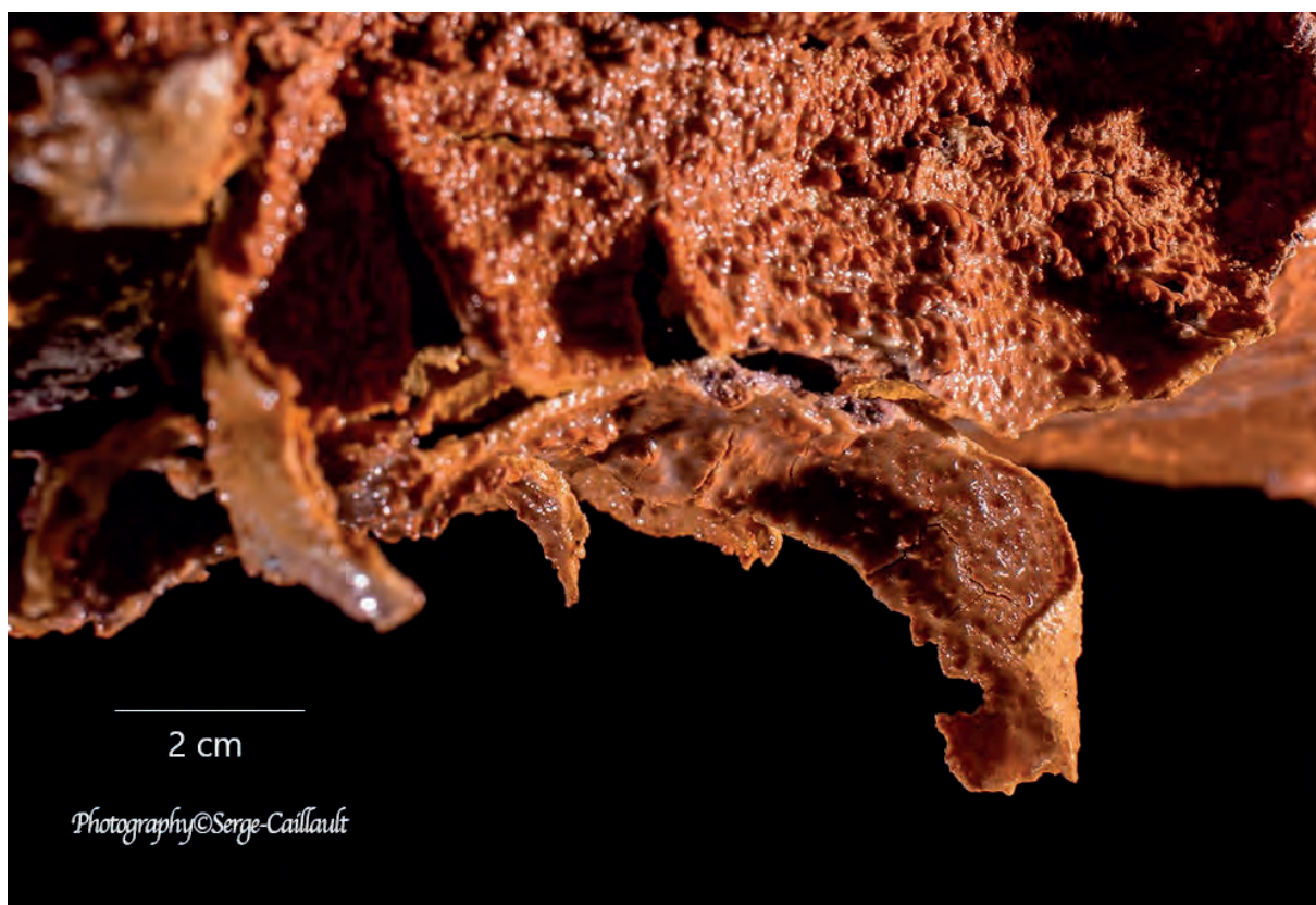
Figure 4: Alterite crisps, centimetric in size, partially detached from the surface of the wall in the Salle du Palindrome (photo S. Caillault).
