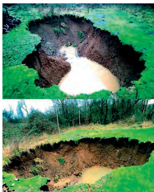
Figure 6: Suffosion in Mečenčani near Petrinja after strong earthquake 29 th December 2020
