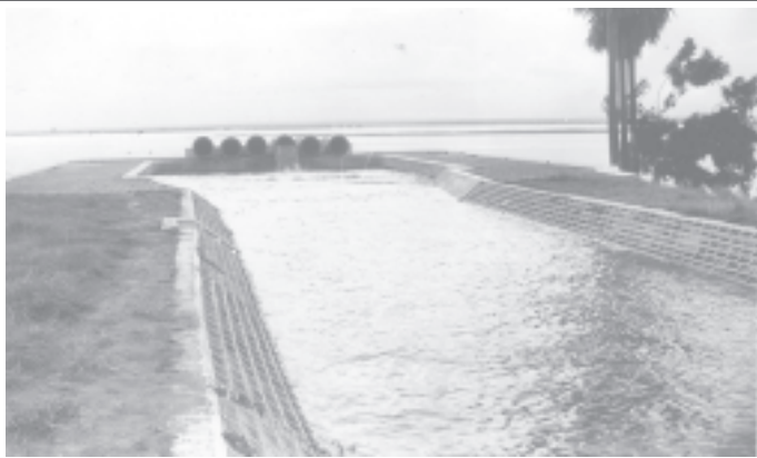
Lt-Gen Ye Myint supervises tasks at Kyawzi River Water Pumping Station Project near Kyawzi Village, Taungtha Township.—MNA
