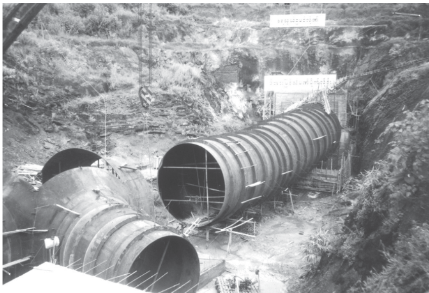
Minister Col Zaw Min inspects Khabaung Hydropower Project. — ELECTRIC POWER NO 1
