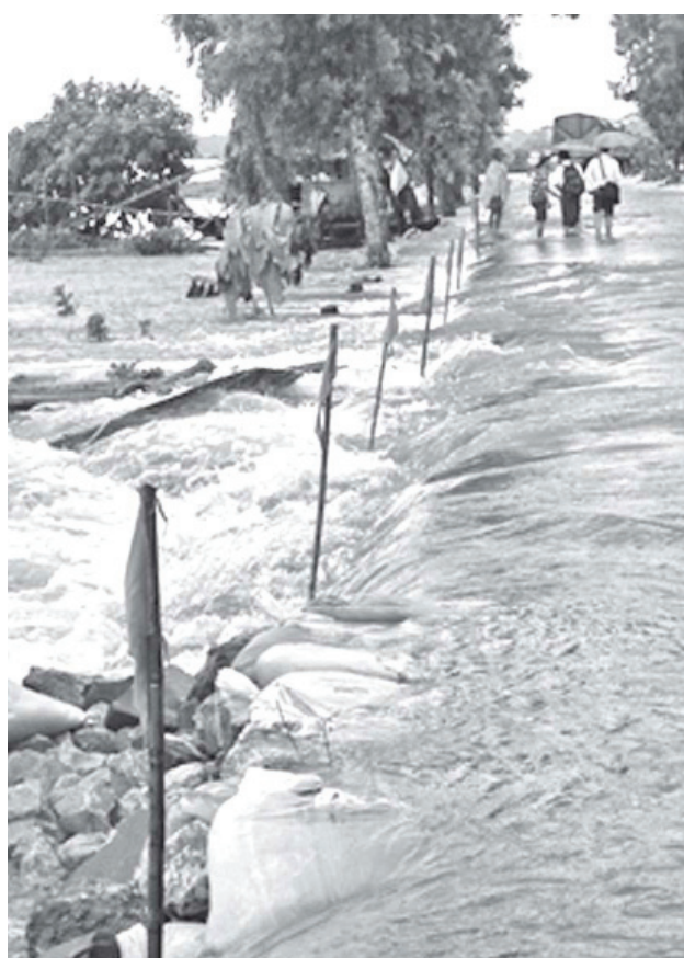
The road section on Yangon-Patheingyi road near Daka Village-tract in Kangyidaunt Township was flooded recently.—KYEMON
