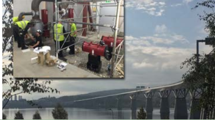
The Sundsvall Bridge in northern Sweden. Inset: Actuator installation in progress
