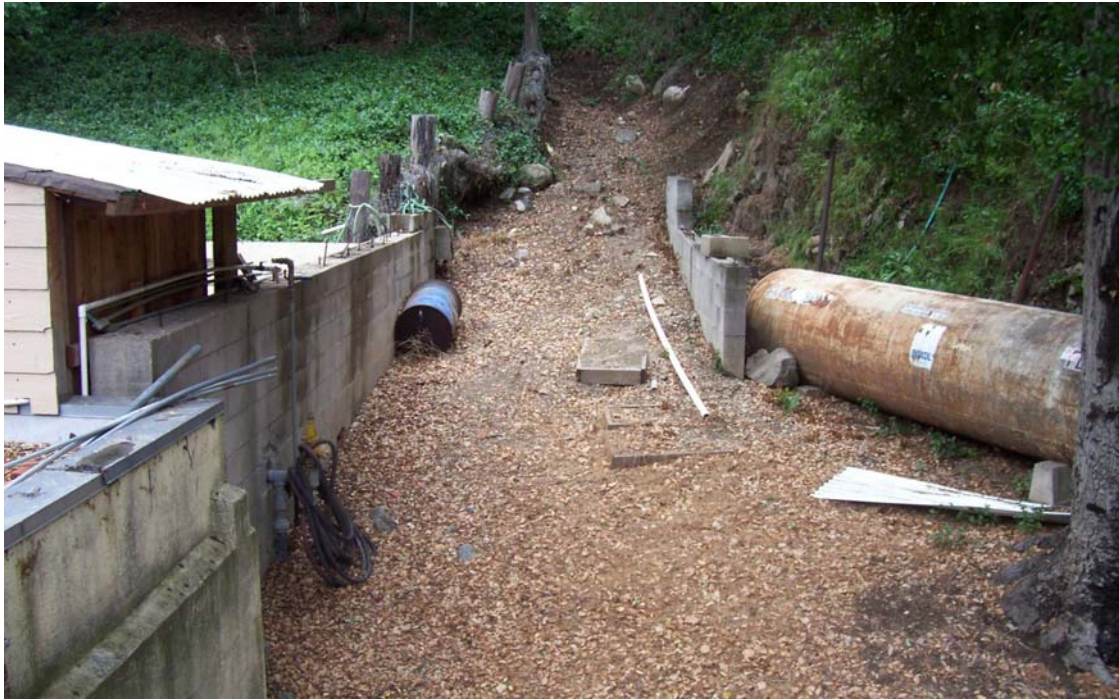
Figure: Drainage Looking Up The Hill
