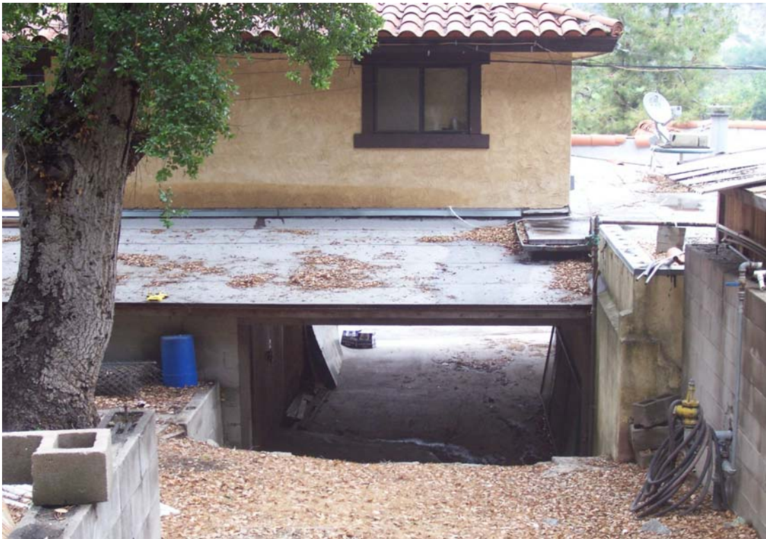
Figure: Drainage Looking Through Carport
