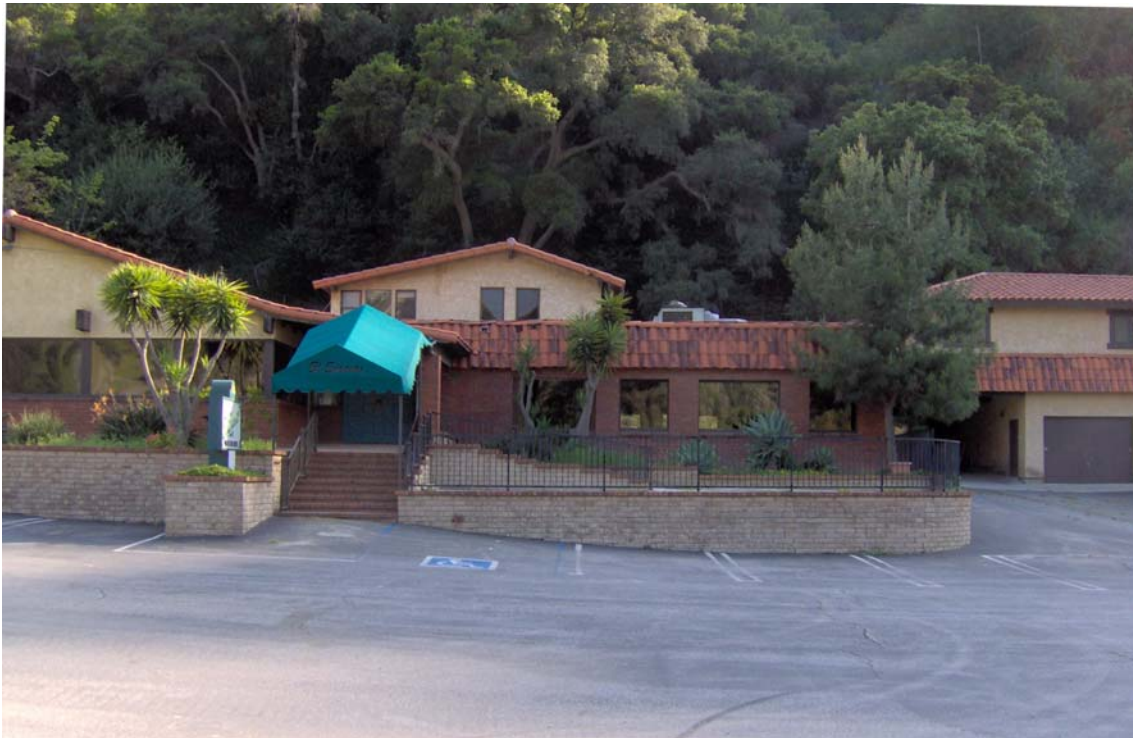
Figure: Existing Restaurant
