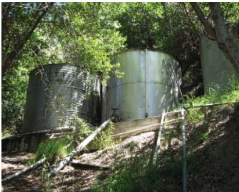
Fig. 4.31 Water well on far side of river
