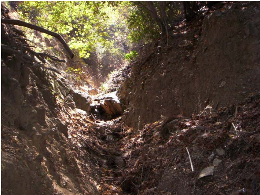
Figure 8: Steep drainage channels behind buildings are cutting deeply into the local historic landslide sediments. Remobilization of these deposits is the primary origin of mud and debris flows surrounding the buildings.
