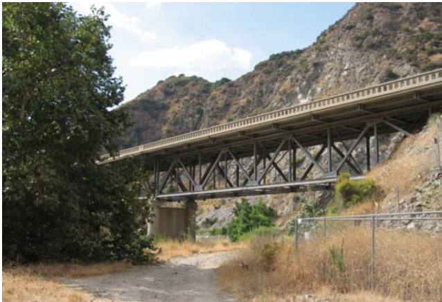
Fig. 4.19 Route 39 Bridge over the San Gabriel River
