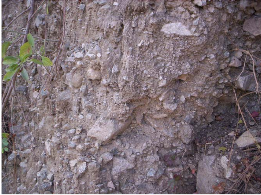
Figure 9: Angular matrix-supported landslide deposits underlying the mobile home park and lower slopes surrounding the buildings.
