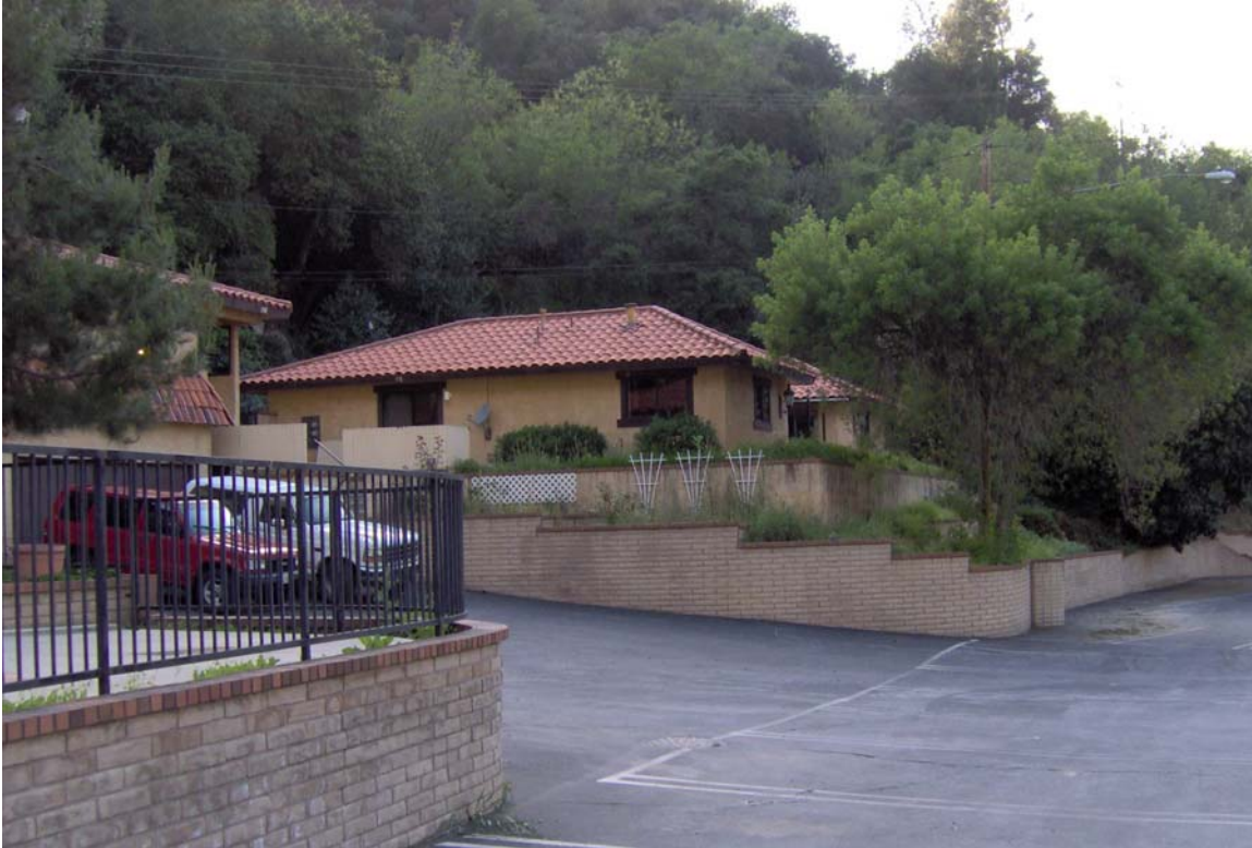
Figure: Existing Two-Unit Apartment
