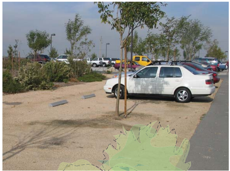
Fig. 6.8, bottom left Detention micro-basin allows stormwater to soak into the soil
