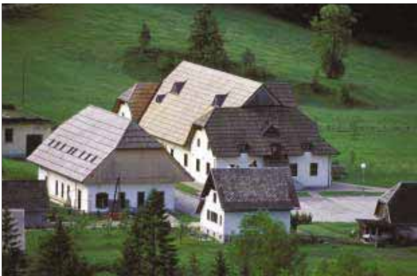
Figure 189. Information Centre of the Triglav National Park at Log in Trenta. Information and education centres in protected areas are playing a crucial role in the conservation of natural values and in raising public awareness.
