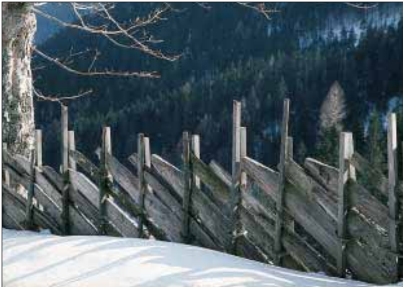
Figure 183. A fence typical of the Topla valley is made of wood off-cuts.
