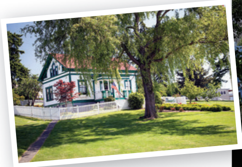
The 1903 keeper's cottage at Tacoma's Browns Point Light Station has been restored and updated with modern amenities.
