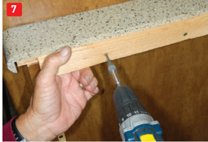
(5) Rubber gas lines are susceptible to damage caused from protruding staples and screws, so be sure to keep them out of harm's way. (6) When working with wood exercise patience. Cabinet modifications will need to be made, and there is not much room for error. (7) The SMEV is roughly 1½ inches narrower than the original range, thus requiring a spacer board to be installed on both sides of the cabinet to fill the gaps. (8) Both spacer boards required sanding for a precise fit.
