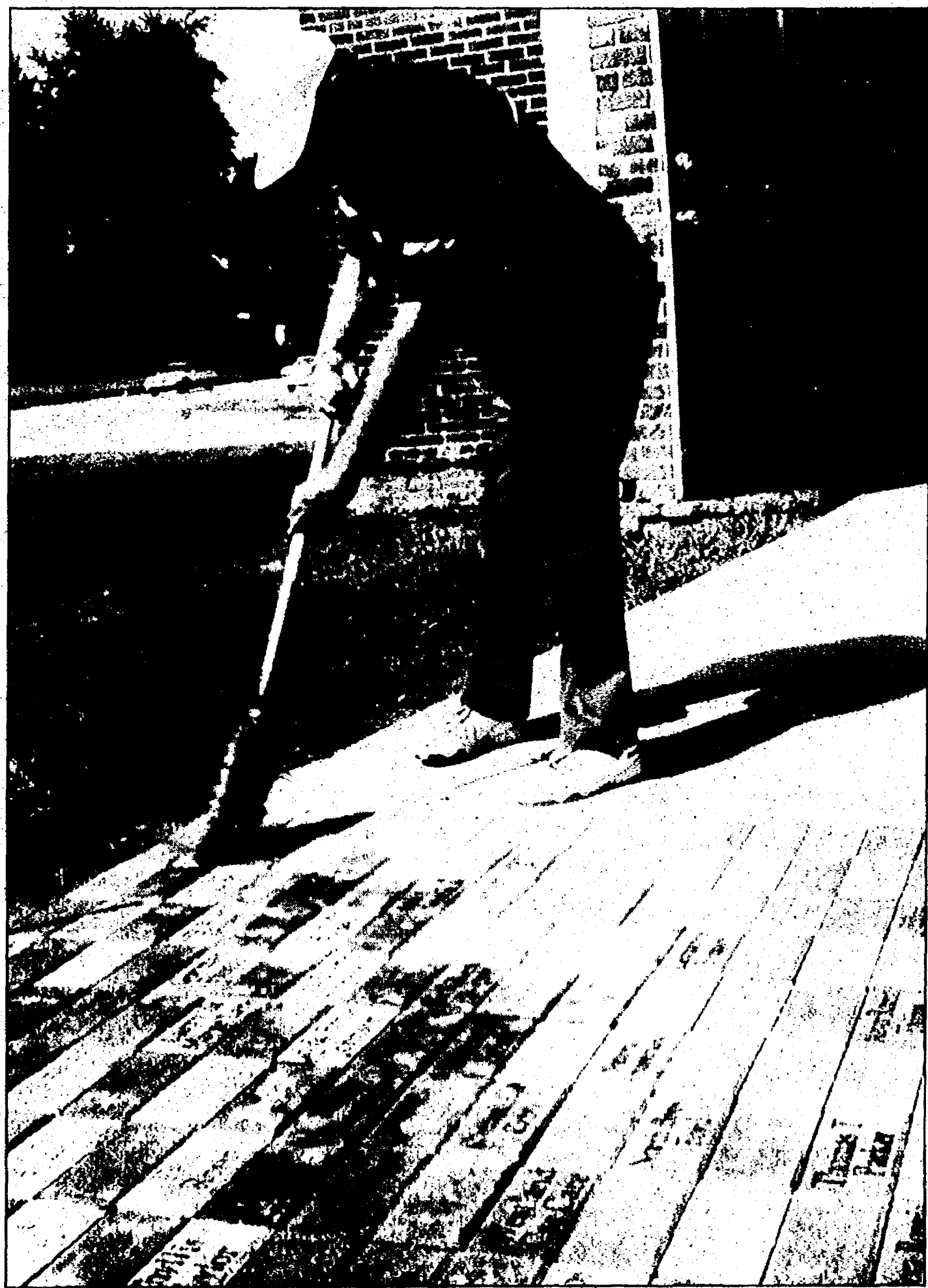
Clean sweep: Ernie Johnson sweeps the brick dust from the newly-installed brick walkway in front of the Perrinsville School entrance.
