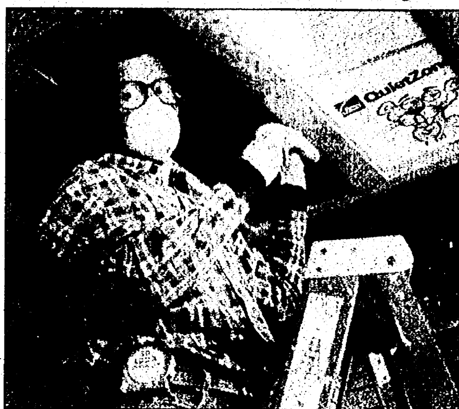
Making it quiet: Dean Johnson, host of public television's home-improvement show, HomeTime , installs Owens Corning's QuietZone Acoustic Batt in a home theater construction. Installing acoustic batts in the frame cavities of interior walls and ceiling/overhead floors in one of the easier ways to control noise in a home theater.
