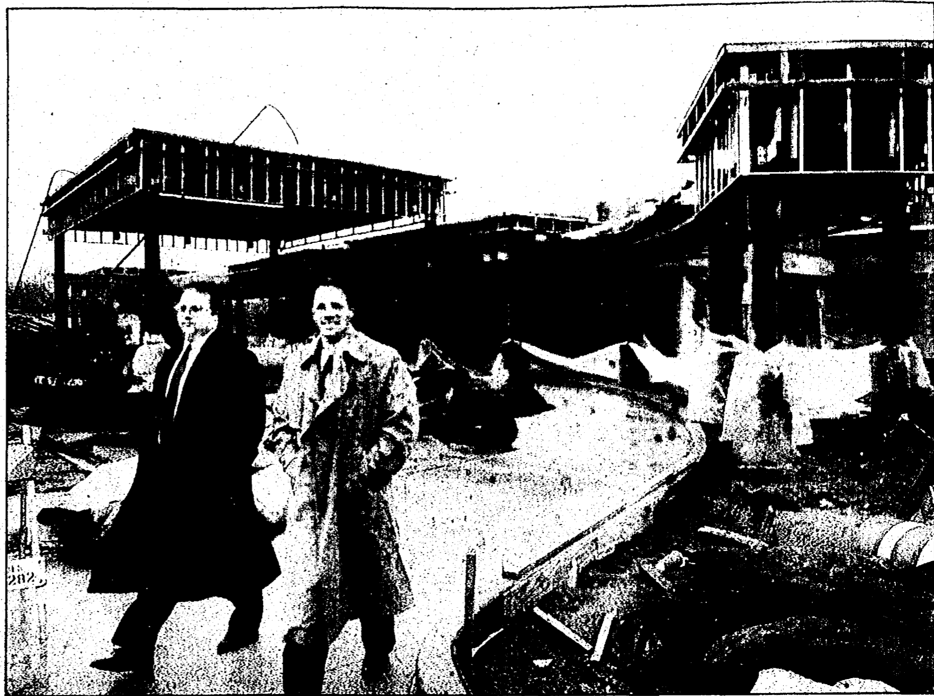
Coming soon: Garden City Hospital staffer Matt Heffner (left) joins facilities director Charles (Chip) Riddle for a stroll along the entrance to the new emergency room. Patients can be dropped at the door under the covered entrance. Riddle expects the new entrance and emergency room to be open next month.
