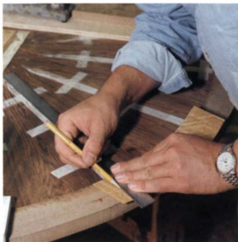
Mark and cut seams. While holding the crossbanding firmly in place, mark seams by lining up a straightedge on the sunburst seam.
