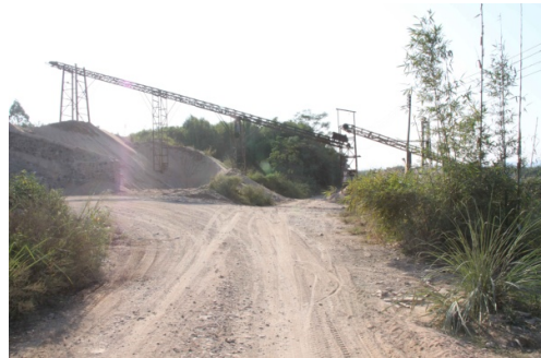
Figure 26. Dredging sand at site 1 in Zhoutian (Zhenjiang River)
