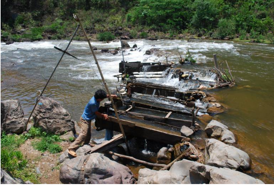
Micro-hydropower generators near Cu Pua village © Fraser Sugden
